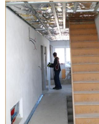
The original design anticipated that the attic could be used in this way; the floor was laid, plumbing and electrical services were extended into the attic during the main construction phase. A major challenge will be replacing the provisional wooden staircase with one that satisfies fire resistance standards.
